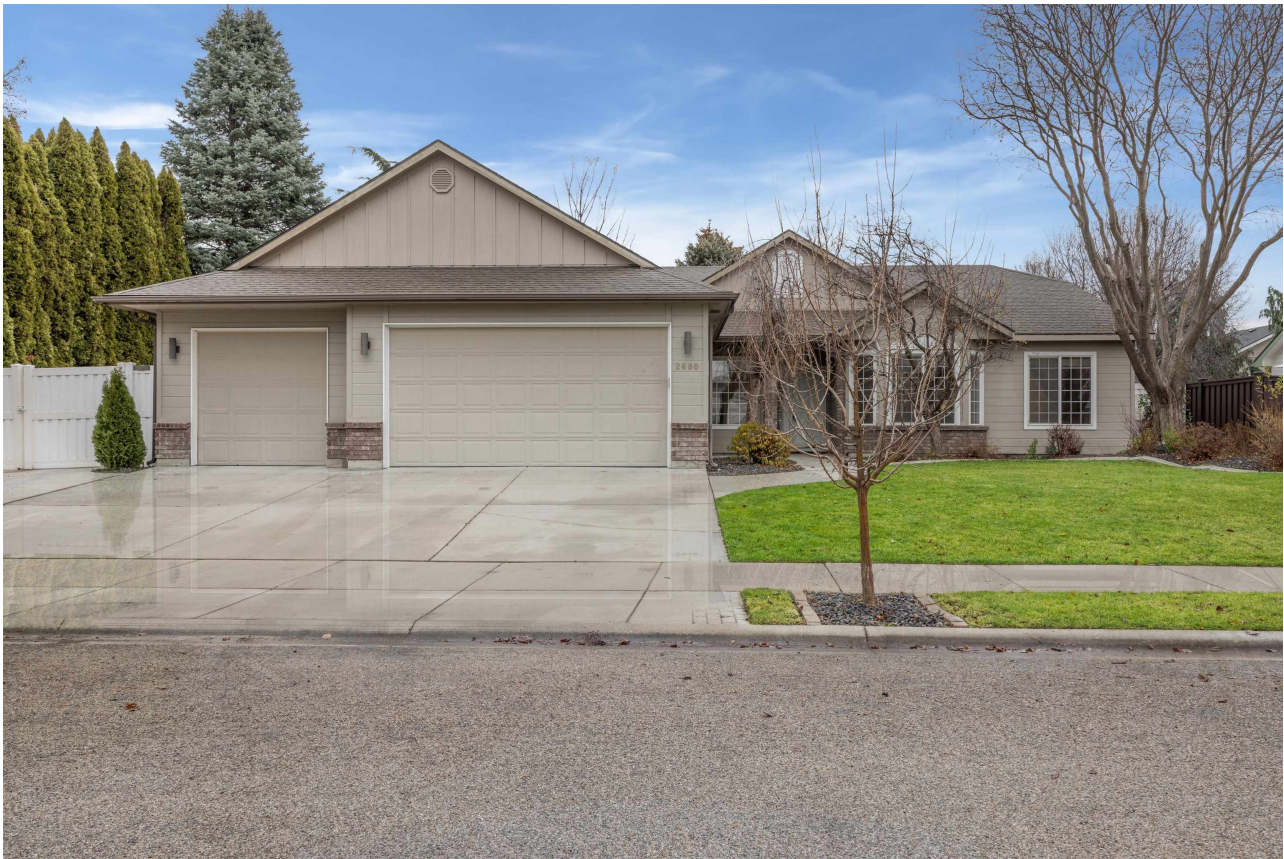
Front Of Structure
